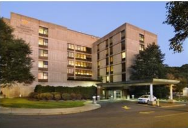
Hebrew Rehabilitation Center Roslindale, MA
